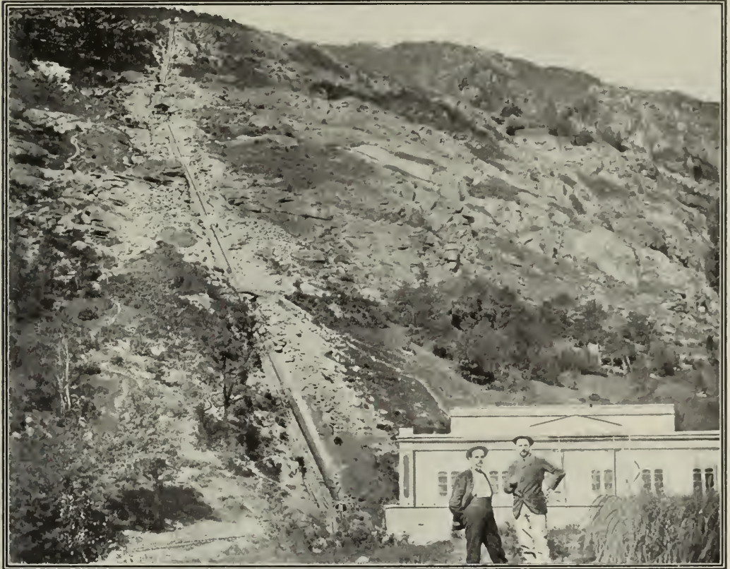
THE PENSTOCK, AND PART OF THE POWER STATION.
